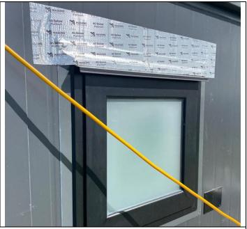
**Next action:** Tape the left side window as this smaller one has been. If successful fit permanent flashings.
