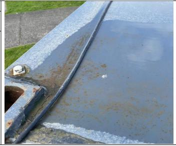
**Next action:** These areas should be cleaned with spirits and sealed. The fixings should be loosened so that silicone can pass to the thread and a new EPDM rubber washer fitted to ensure a good seal. We would need to remove one of thee to investigate what the fixing is etc.
